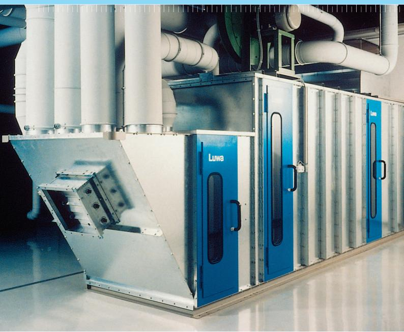
Centralized air handling system for textile and nonwoven applications
