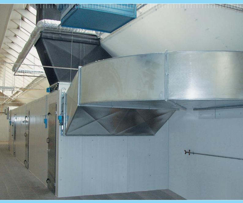
Sandwich panel housing for centralized air treatment systems for textile and nonwoven applications
